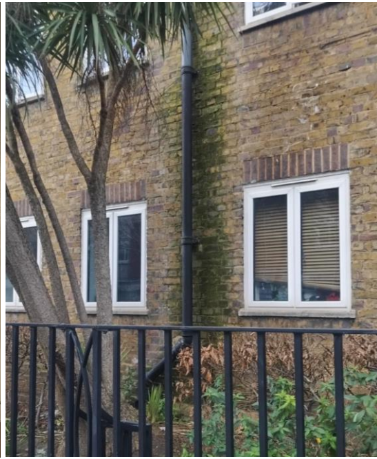
Left: Evidence of Abdul's leak in his daughter's bedroom. Right: Moss growth on brickwork caused by leaky gutters at a property in Maude House.
