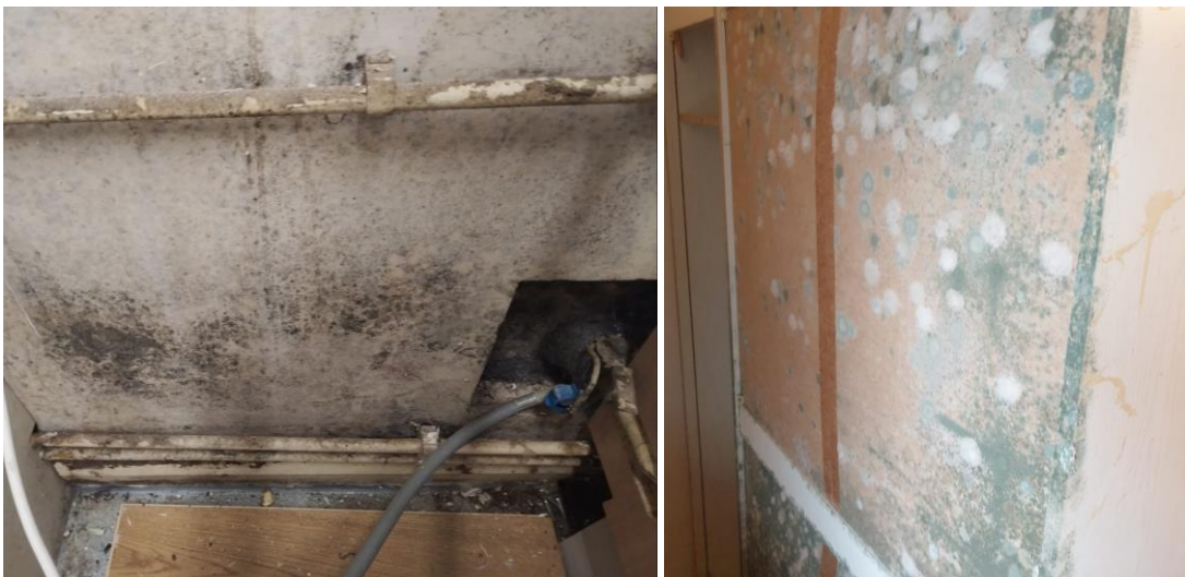
Left: Example of condition of property in a flat in Jellicoe House after repairs to address mould. Right: Back of wardrobe in a home in Sturdee House.
