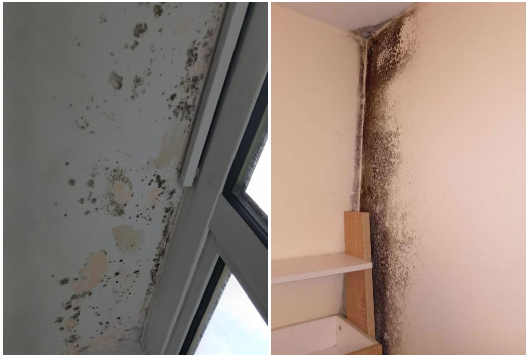
Left: Example of mould around a window area in a flat in Haig House. Right: Example of Mould in a bedroom corner in a Flat in Jellicoe House.
