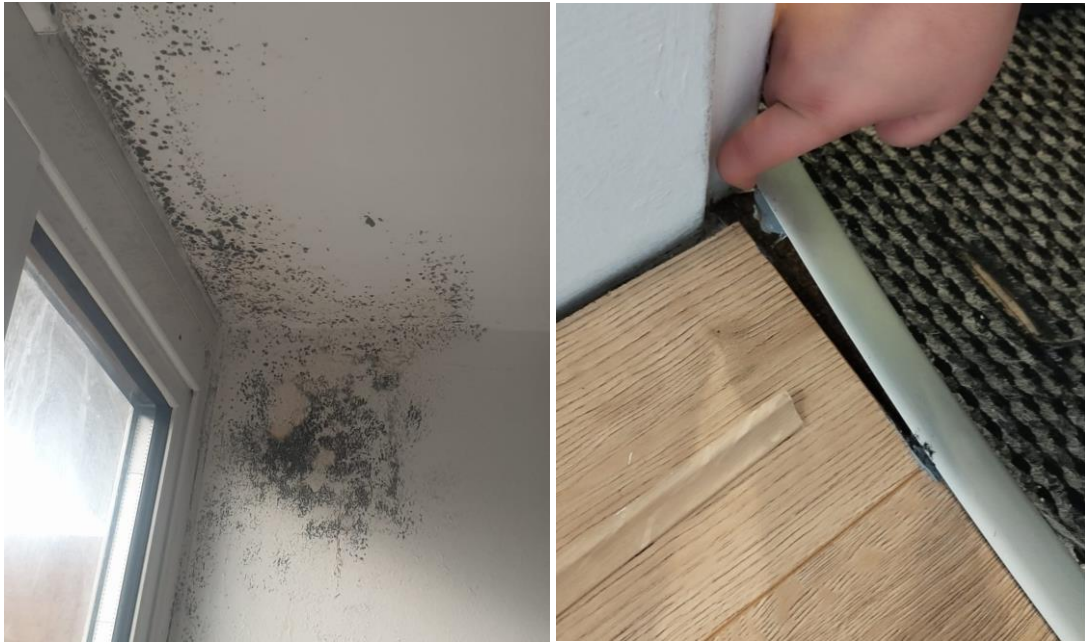
Left: Example of mould around a window in Sturdee House. Right: Example of poor repairs in a flat in Haig House following repairs.
