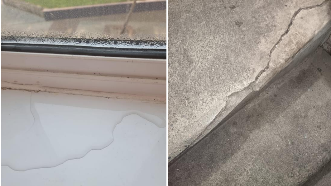
Left: Example of condensation on windowsills in Haig House – widespread problem in the Nags Head estate. Right: Example of crumbling stairs at Sturdee House – several incidents have been reported as a result of this.
