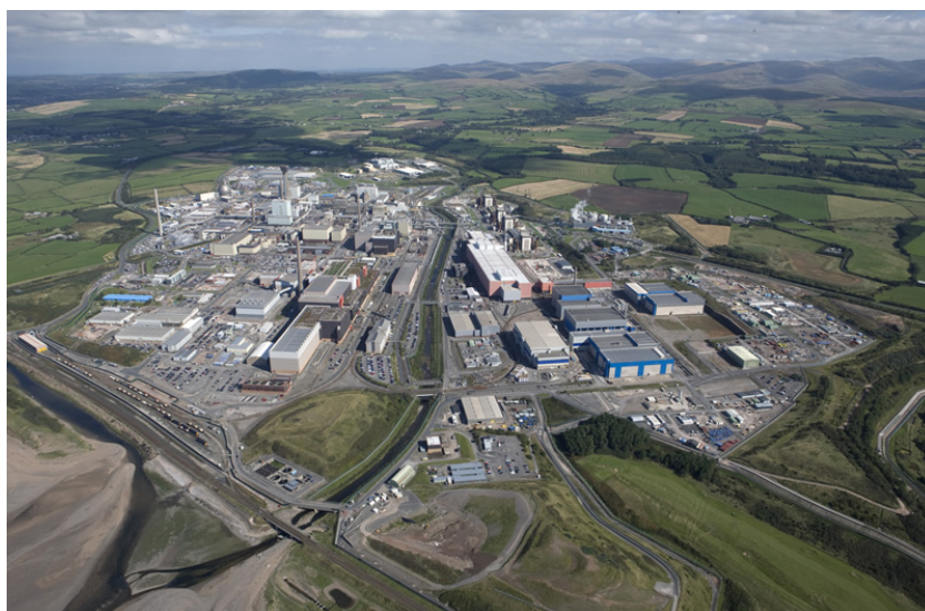
Aerial view of Sellafield (Photo: Sellafield Ltd)
